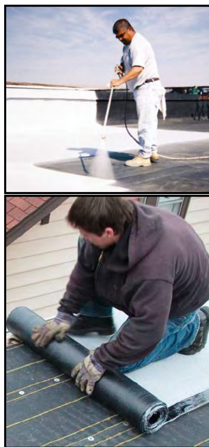
Figure 6: Two Cool Roof Installations
